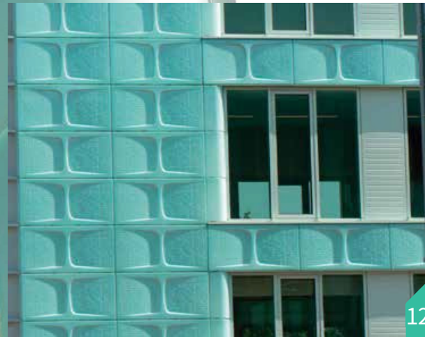
11 Philips Science Park Wall Cladding LEXAN™ SG305 SLG sheet
