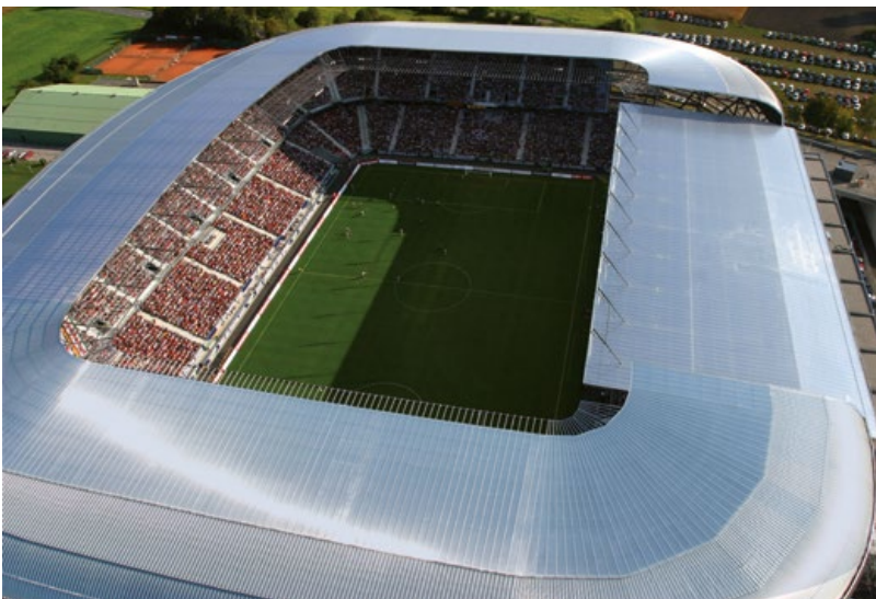
Wörthersee Stadium Roofing. Roof is made of transparent LEXAN™ THERMOCLEAR™16 mm sheet.
