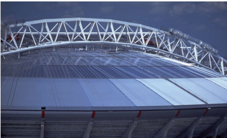
Amsterdam Arena in Amsterdam, the Netherlands is Europe's first stadium with a sliding roof, made from LEXAN™ THERMOCLEAR™ transparent sheet. 20.000 m 2 - The sliding roof was necessary to allow events to be staged regardless of the weather.
